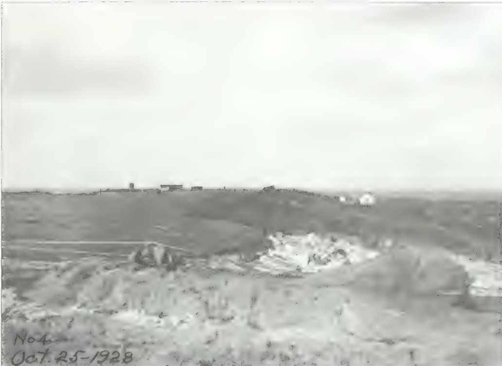
Figure 5.5. Sand being hauled into place in front of the terreplein, Nine Gun Battery, 1928. Engineers covered the concrete structures with sand and earth for concealment and to help absorb the impact of enemy fire (GATE 7009).
